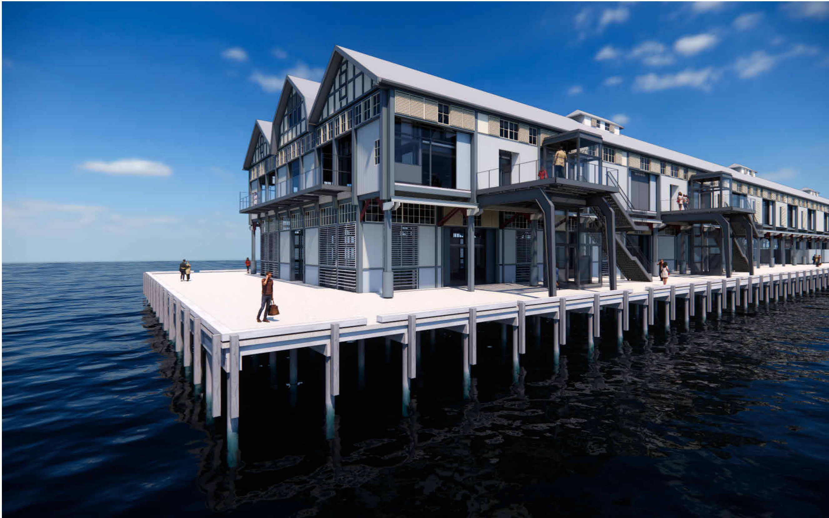
1. North west view of Pier 9.
