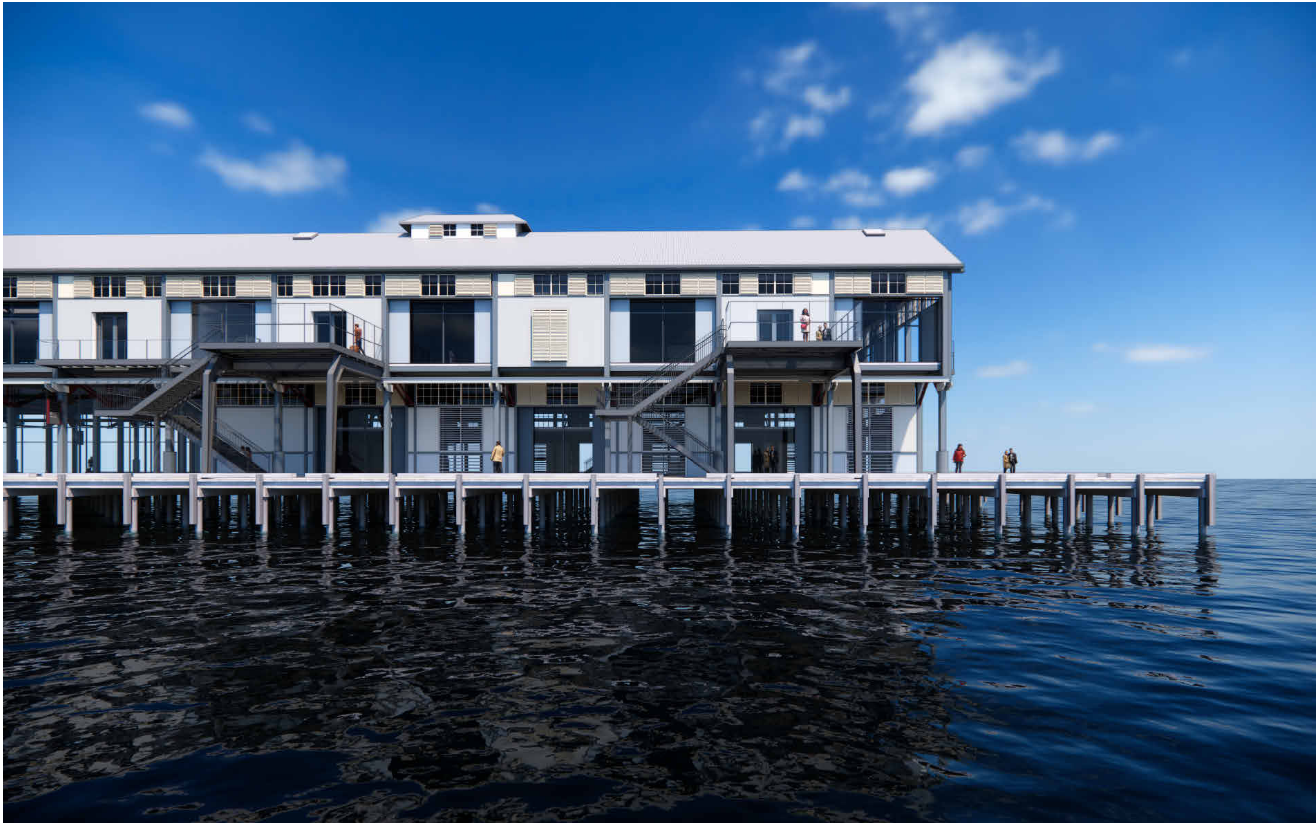
2. Eastern view of Pier 8.
